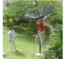
CATHALAC/SERVIR Antenna Installation
